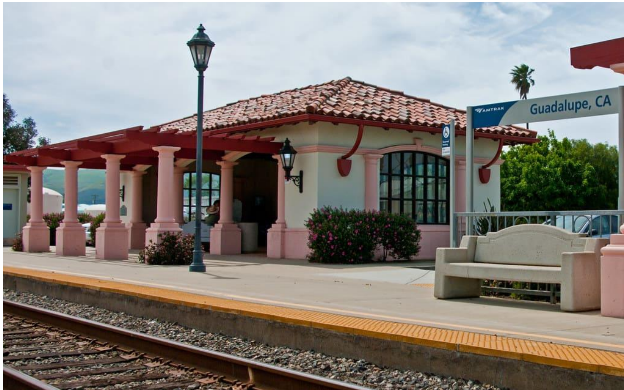
Guadalupe Amtrak Station (GUA). Credit: Amtrak.
