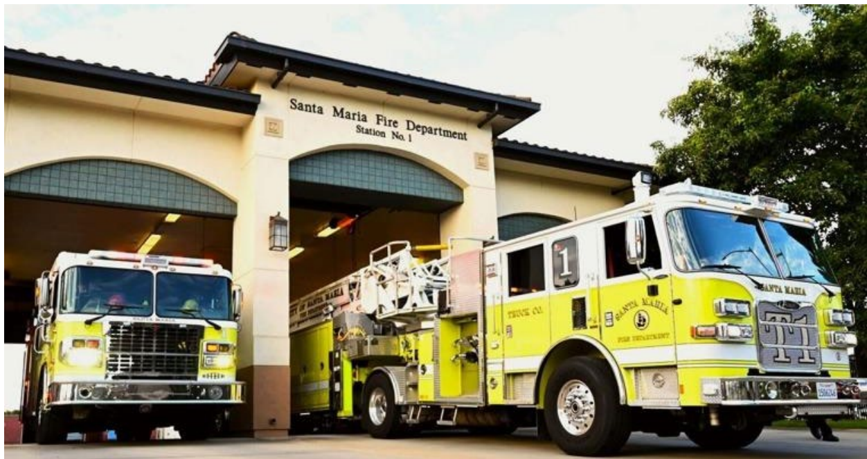
Santa Maria Fire Department Station No.1. Credit: Randy De La Peña
