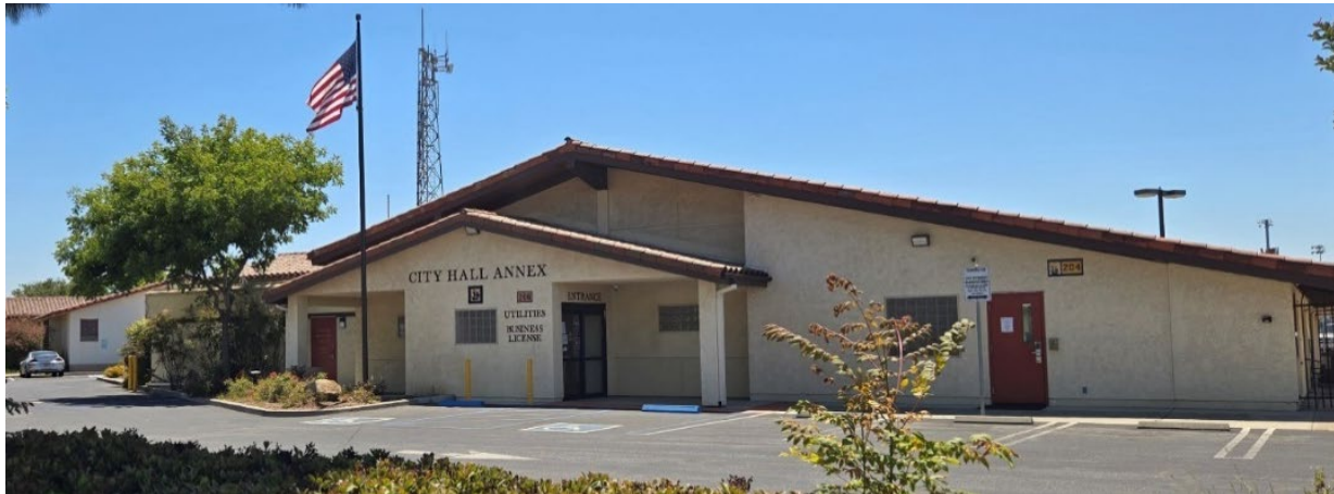
City Hall Annex building located on Cook Street.
