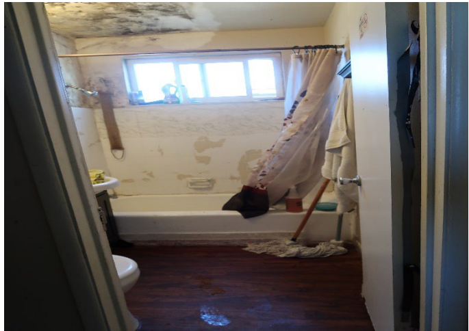
Examples of building code violations and substandard housing conditions include unpermitted construction of a shed used as a dwelling unit and extensive mold in a bathroom.
