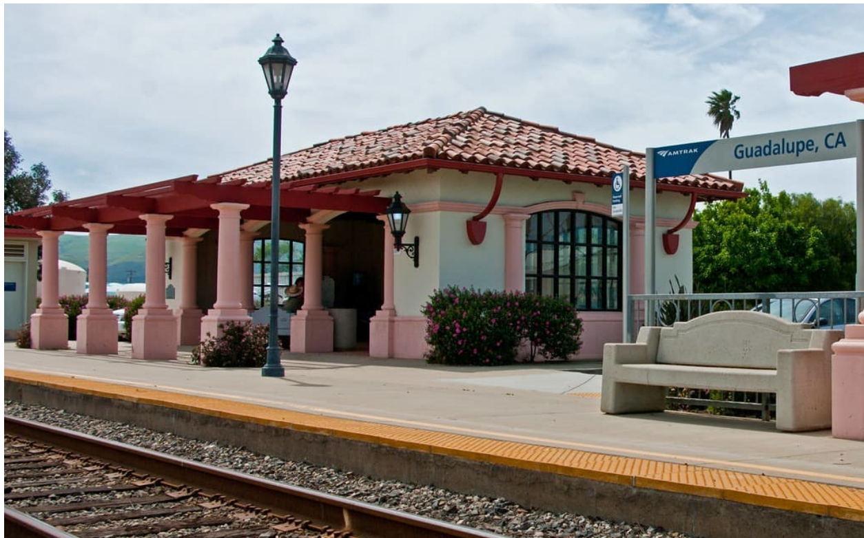
Guadalupe Amtrak Station (GUA). Credit: Amtrak.
