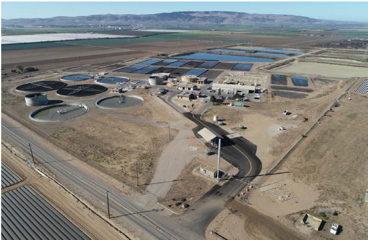
City of Santa Maria Wastewater Treatment Plant.
