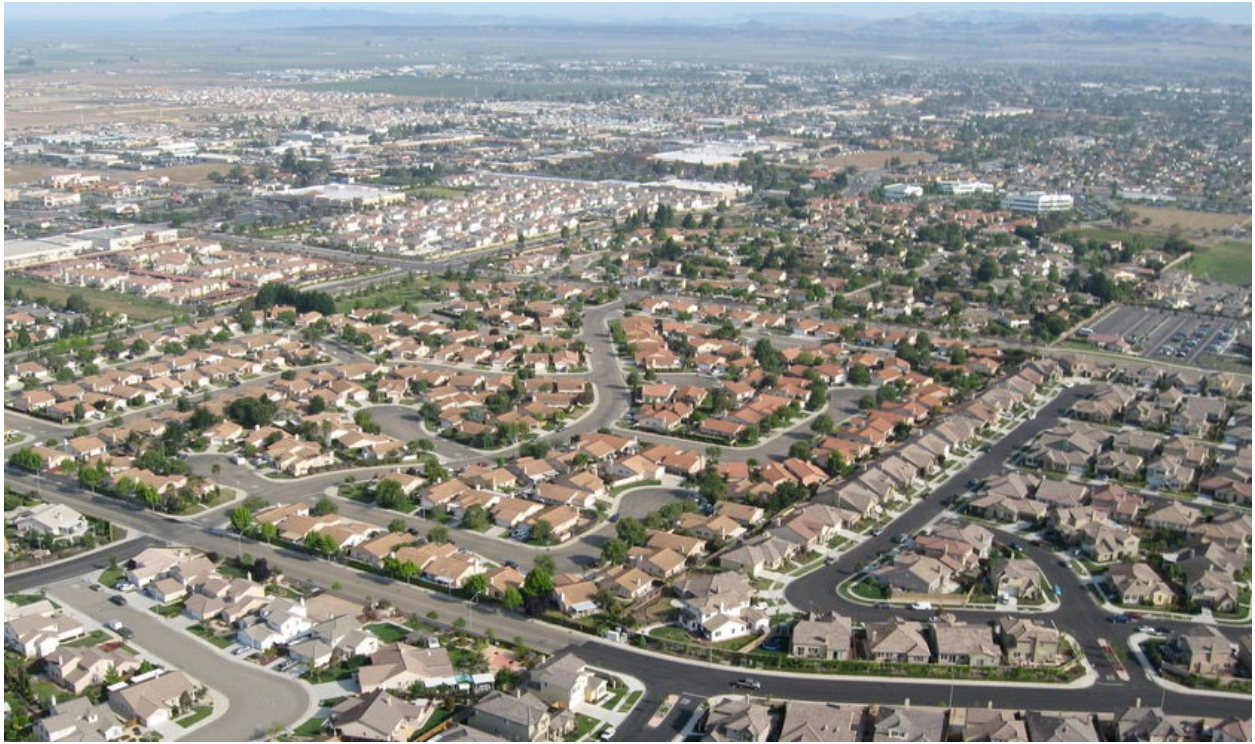
Single-family residential subdivision in the southern part of the city.
