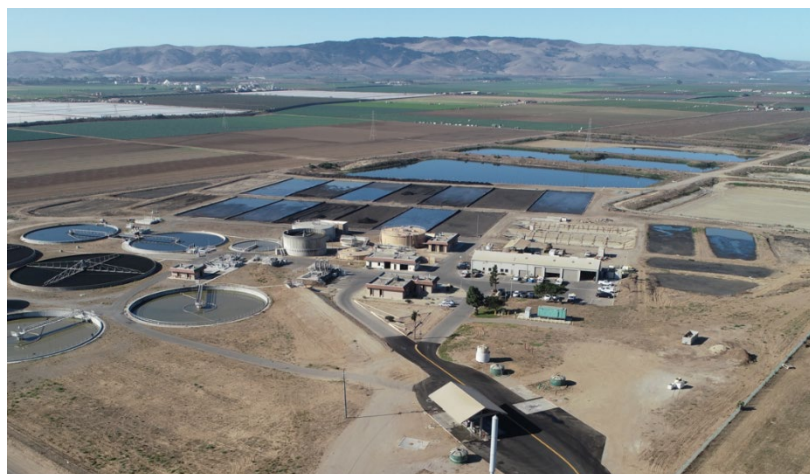
City of Santa Maria Wastewater Treatment Plant.
