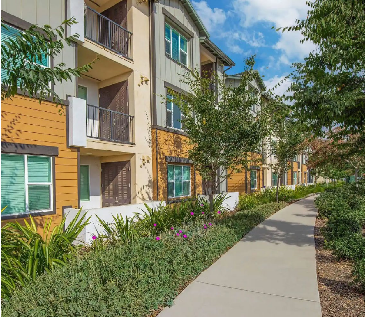
A multi-family apartment complex in Santa Maria.
