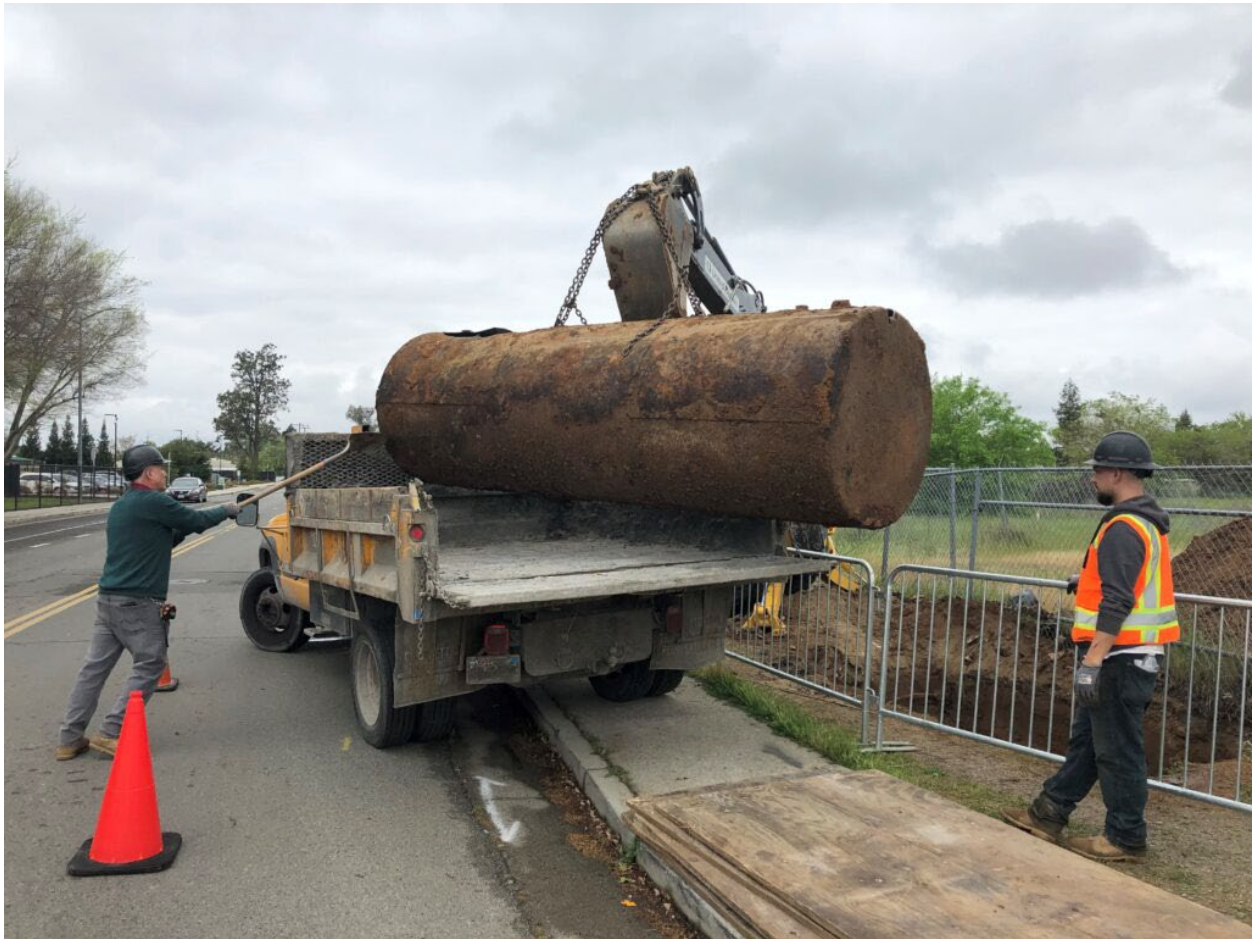
An abandoned underground storage tank is removed as part of the remediation process.
