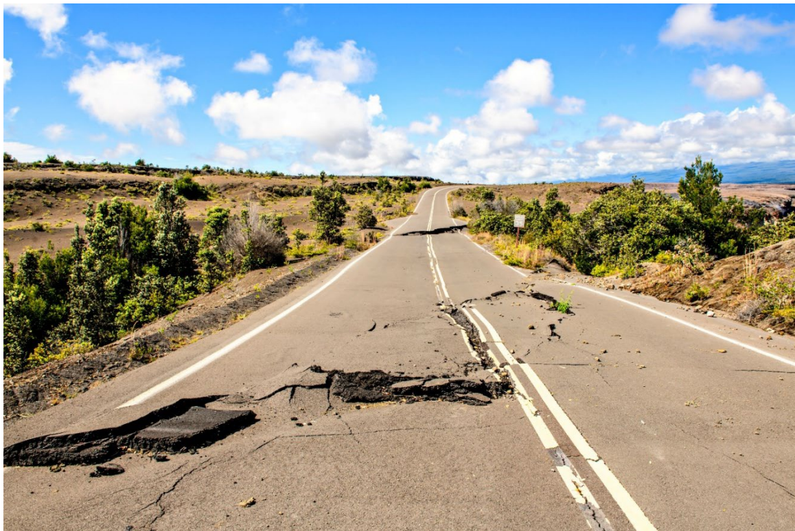
Earthquake causes major damage to roadway.
