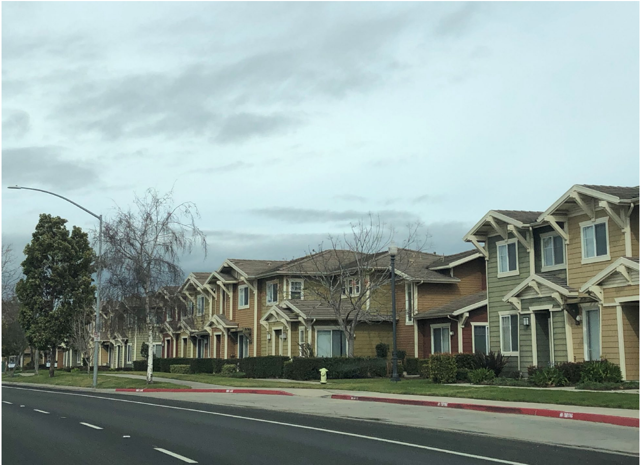
Housing abutting main corridors is often impacted by transportation noise.
